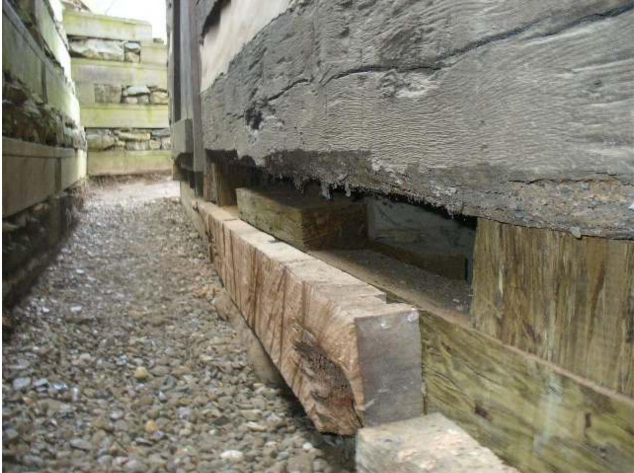
The manufactured beam in place supporting the rear logs with a trial veneer.
